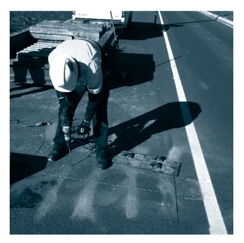
In early June, 2012, SGS accepted a contract from Macmahon of Australia to provide complex pavement engineering services for an asphalt beam recovery project in Perth. From mid-June until late July, SGS experts performed pavement and sub-grade testing investigation services using state-of-the-art testing methods which included deflectometer laser profiling, falling weight deflectometer technology, the South African deflectometer cone penetrometer method and geotechnical analysis.
